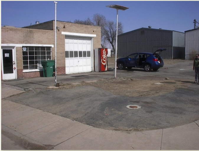
The Town of Milliken successfully redeveloped a former gas station into the Milliken Police Station. The new building improves the effectiveness of the community's policing efforts, which represents a socially sustainable service delivery model.
