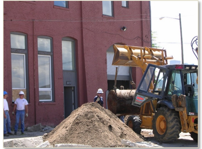
The Source is a 19th century steel refinery that was repurposed to house a group of local Denver breweries, eateries and specialty grocers. The reuse applied sustainable building practices.
