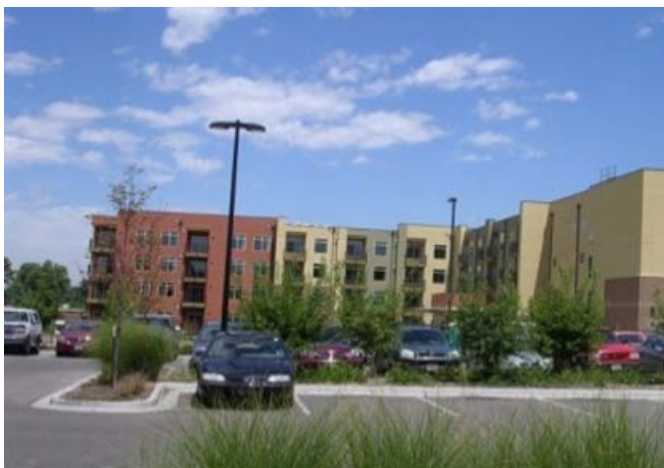
The redeveloped Dahlia Square in Denver's Park Hill neighborhood provides affordable housing and medical facilities.
