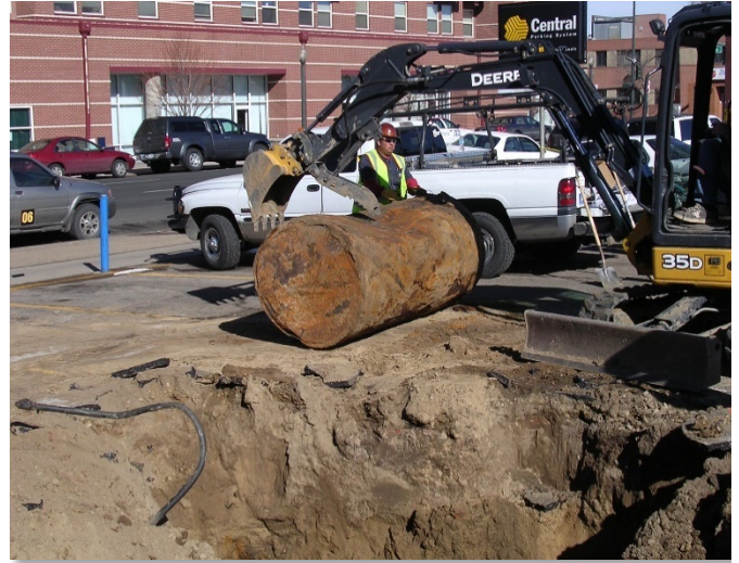
The Redevelopment Fund can provide financial and technical assistance for removal of a petroleum storage tank from the property.
