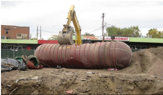
Underground Storage Tank Removal
