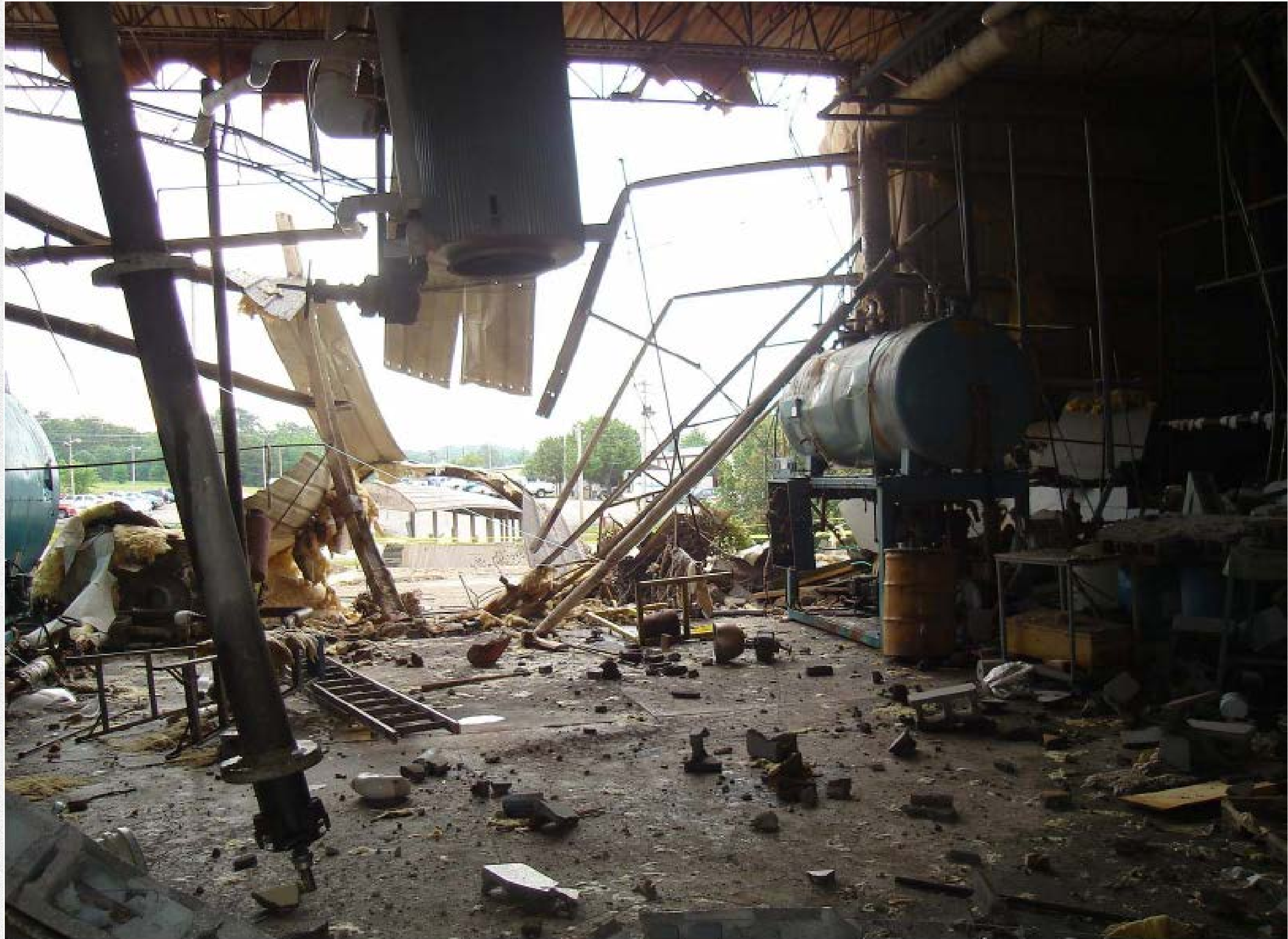
Photo #5 – Knocked Down Exterior Wall Viewed from Inside Boiler Room (East Wall)
