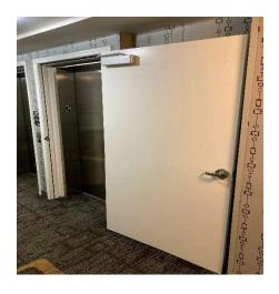
These Smoke Curtains and Smoke Doors would prevent firefighters from visually observing the elevator lobby when in the closed position, so they are **not** ASME A17.1 code compliant.
